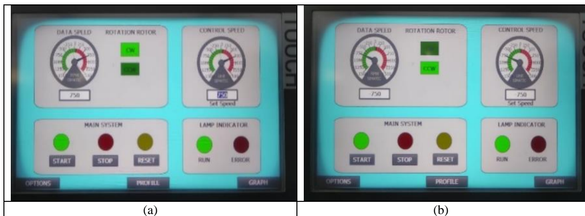
Figure 7. HMI display at first experiment, a) forward operation, b) reverse operation
