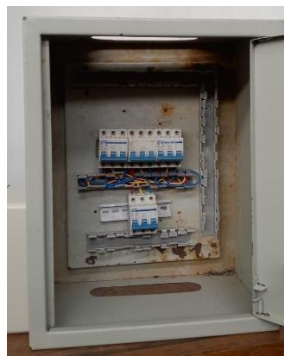
Figure 1. Distribution panel circuit
